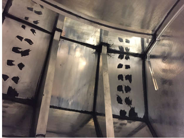
Figure 23: The stressed areas were covered with RTV sealant.
