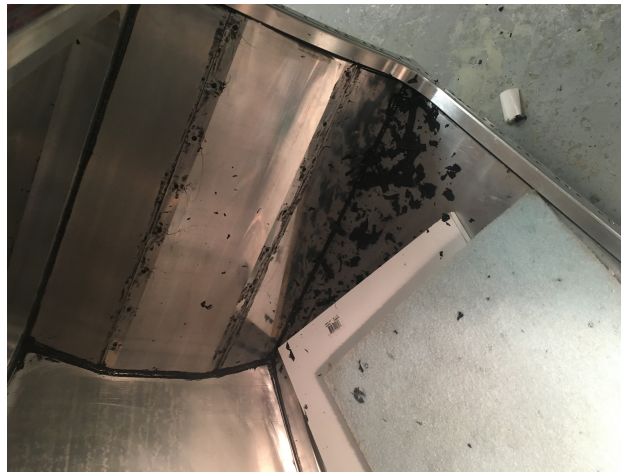
Figure 12: The sealant was scraped off with a utility knife.
