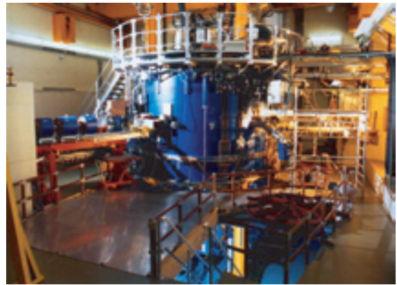
Figure 3.10: A photo of the K=600 MeV, superconducting AGOR cyclotron at KVI.
