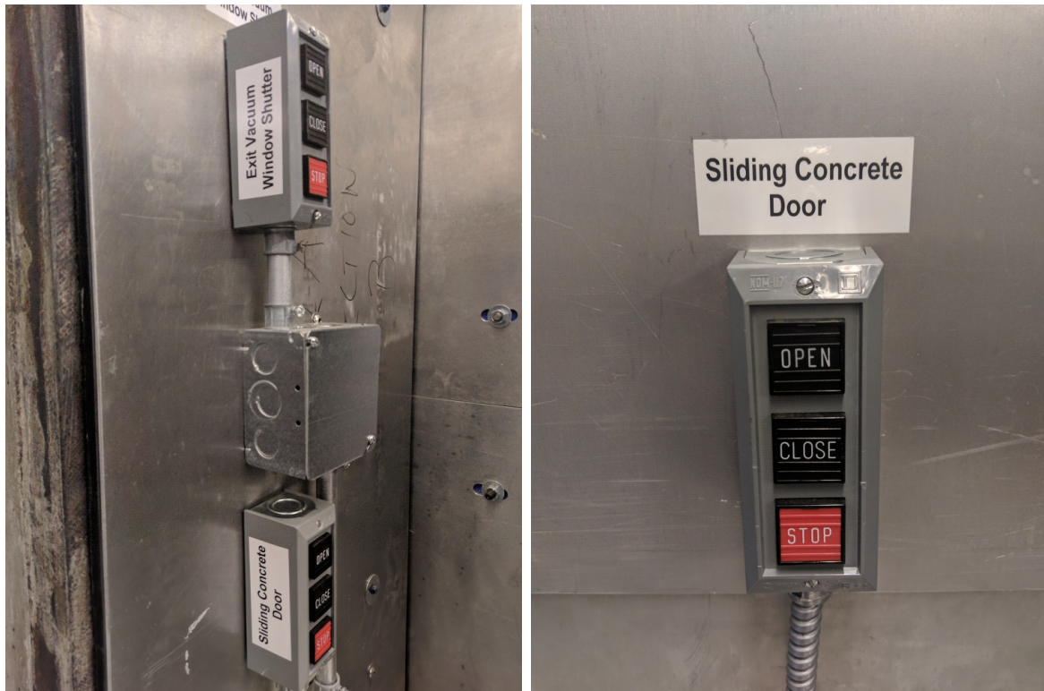
Figure 5.13: SHMS barn door controls. The left picture shows the controls located in electronics hut. The bottom buttons control the barn door and the top buttons control the SHMS vacuum extension shutter. The right picture shows the barn door controls located inside the detector hut.
