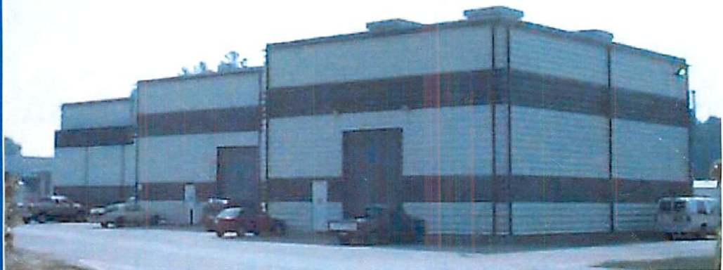
Central Helium Liquefier Complex
