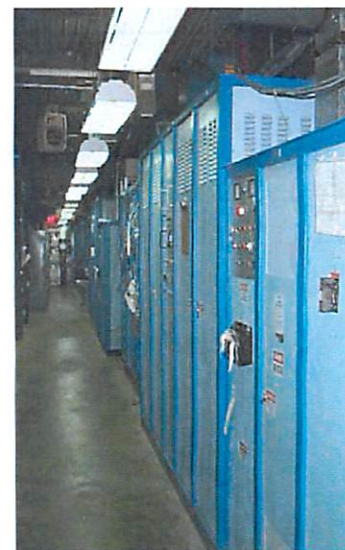
Typical relay rack
