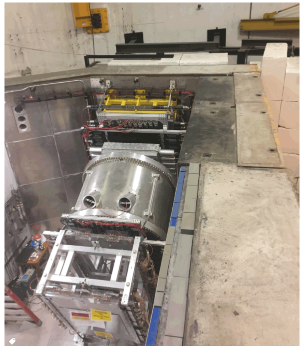
Figure 66: Photo showing a cross section of the Shield House Wall highlighting the layers of custom materials used.
