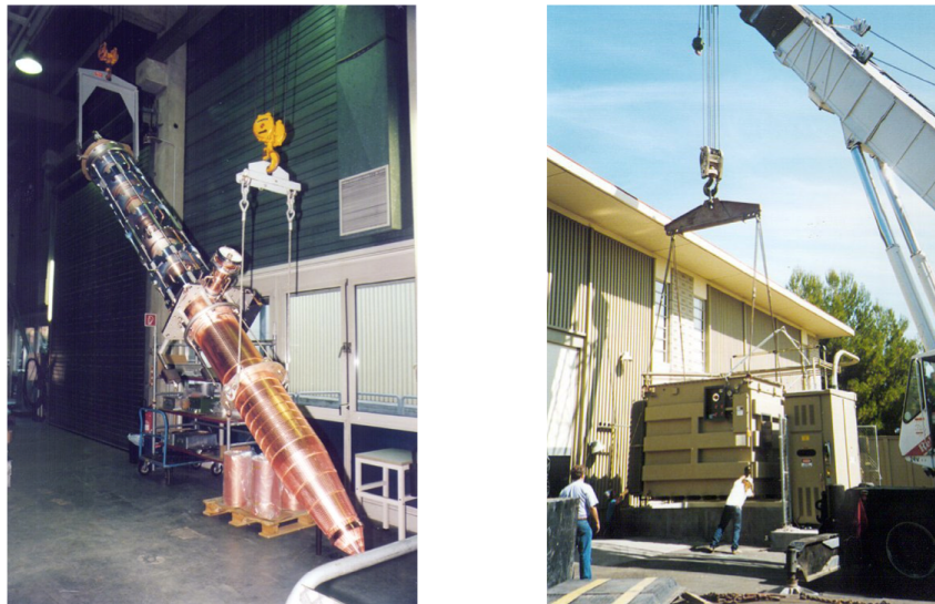
Figure 9.78: PEP-II 1.2 MW klystron and 2 MVA switching power supply.
