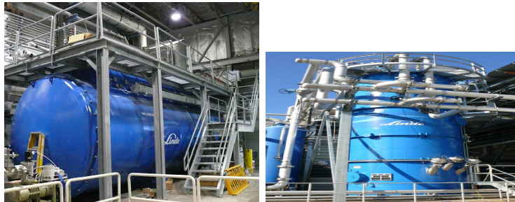
Figure 11.6: 4.5 K cold box lower (left), and upper (right).
